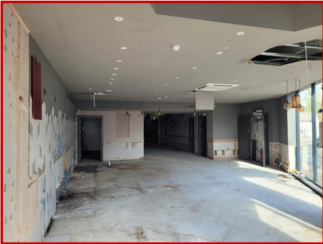
Internal photos of ex Costa – 723a
